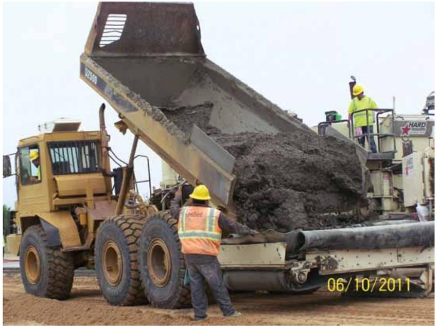
**Off-Road Truck Dumping a Concrete Batch in Reno County, KS**
