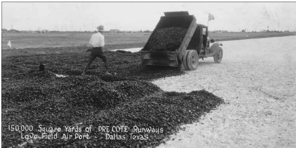
**Figure 2 Laying Asphalt**
