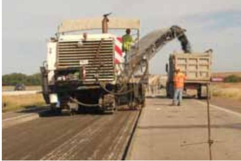
The pavement was constructed in 1964 and consisted of a hot mix asphalt surface and base for a total of 15 1/2". Over its 47 years of life the original pavement was resurfaced and rehabilitated five times and an additional 8.7" of
