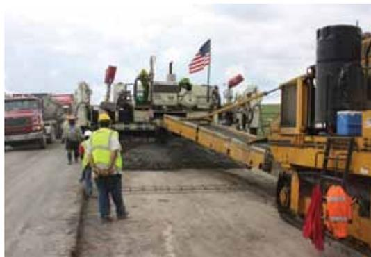
Things became even more exciting as the project got underway. Once the existing asphalt roadway was milled in preparation for the concrete overlay, it quickly became clear that the underlying asphalt pavement would be unsuitable to handle a thin concrete section. Koss and KDOT came together and deemed the
